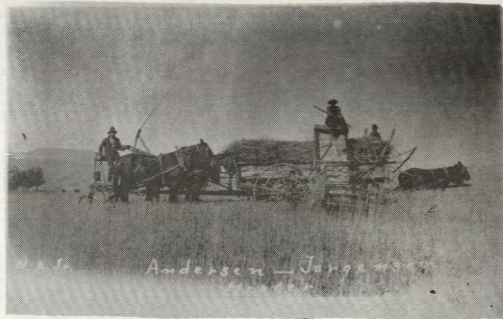
Six men formed a heading crew - the header man, three driving header boxes, a loader, and a stacker.
